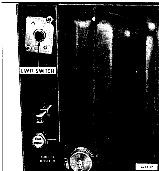
Figure 43—Type II Furnace Limit Switch
