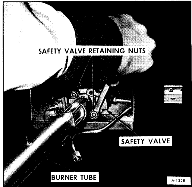
Figure 18—Removing Nuts Holding Safety Valve
