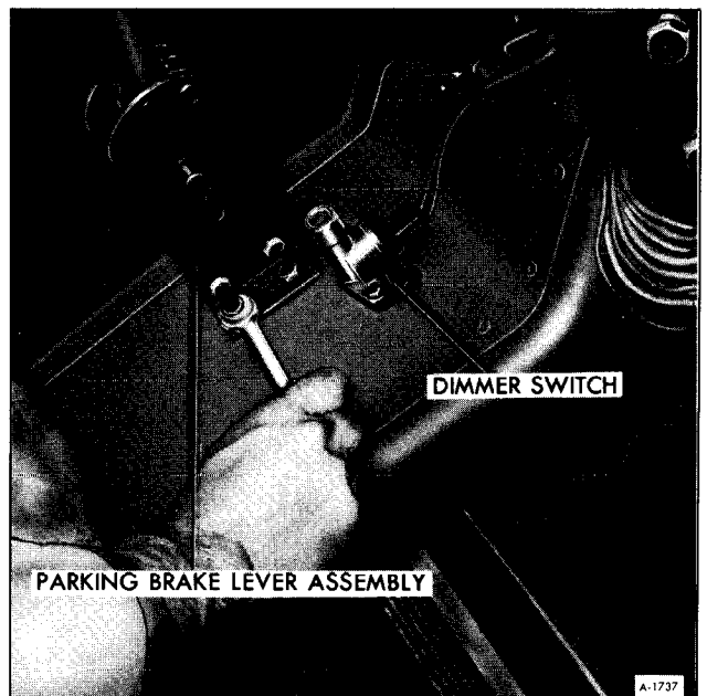
Figure 23—Removing Parking Brake Lever Retaining Nuts
