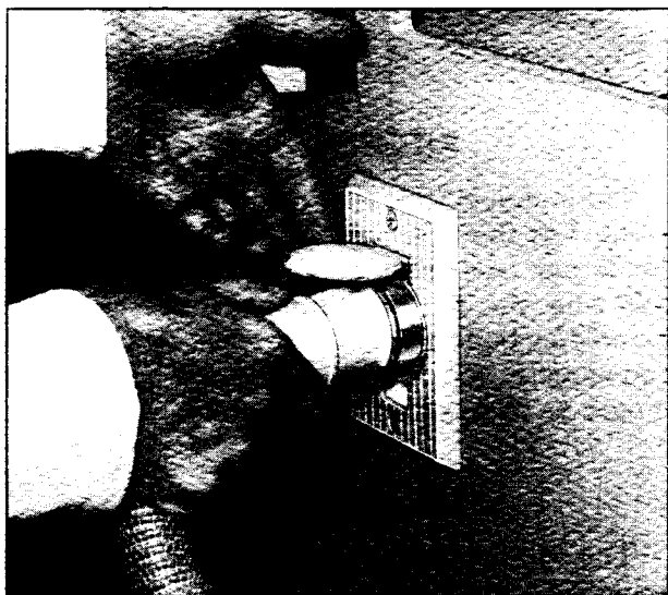
Connecting Flex Hose to Wall Socket (ZEO 6581)
