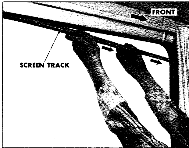
Removing Screen Track
